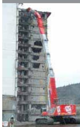
The SK3500D demolition machine has a maximum reach of over 65 meters. The SK3500D is recognized in the Guinness Book of Records as the demolition machine with the longest high reach in the world.
