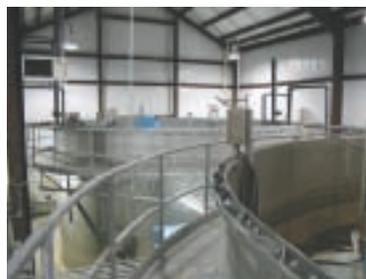
An example of a sequential batch reactor tank operating in Delaware which processes 51,000 gallons of wastewater per day.
