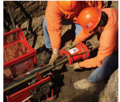
Using a technique pioneered in the UK, our New York business now carries out 'live' gas mains replacement, where the new mains are inserted into the old mains while they continue to operate. We can complete our work more quickly, at a lower cost and with less disruption to our customers and the public.
