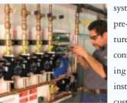
systems. Hydronex panels are pre-engineered and manufactured in three typical modular configurations for radiant heating applications, providing installers with an alternative to custom built panels.
