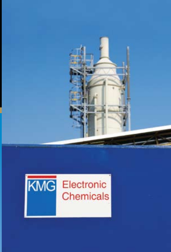
Exterior Shot of Milan Plant
