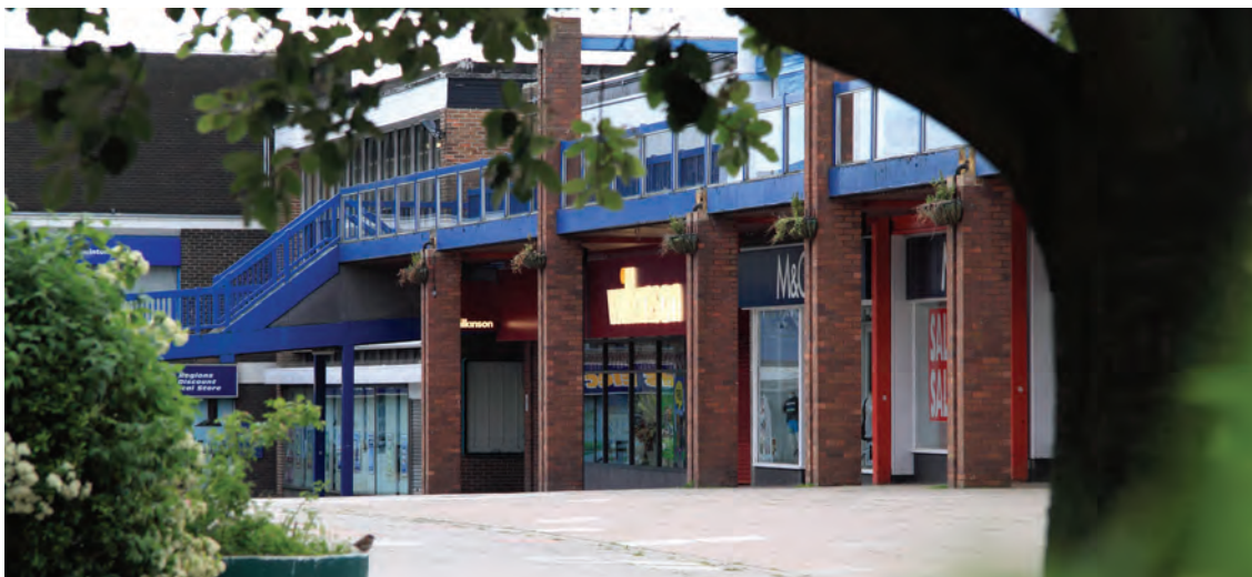
Above, left & below left: Newton Aycliffe Shopping Centre, County Durham
