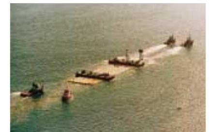
3 Four tugs tow the element into the channel while a global positioning system pinpoints its final position to within a few centimetres
