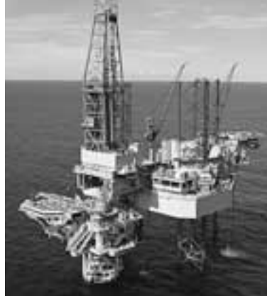
Left: Wellhead platform, Bayu- Undan liquids project. Photograph courtesy of ConocoPhillips Australia Pty Ltd.
