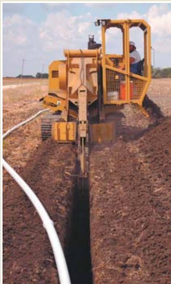
Installing utility lines along a highway.
