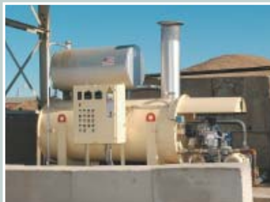
Ready-mix producer in Peoria, Illinois uses a Heatec heater to heat sand stockpiles for mixing concrete during winter.
