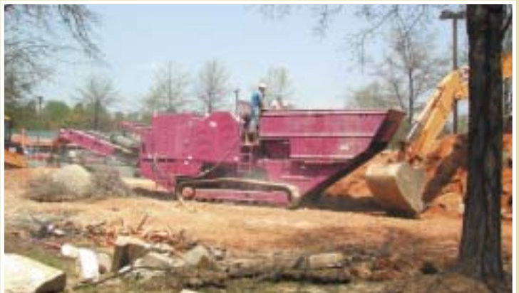
The Pioneer track mounted crusher at a recycling job in the Baltimore area.
