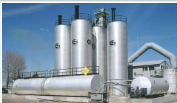
Storage tanks for asphalt, polymer modified asphalt, and fuel oil.
