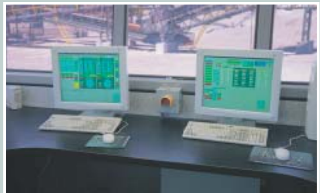
The new TC 2000™ control system operates the plant via PC.
