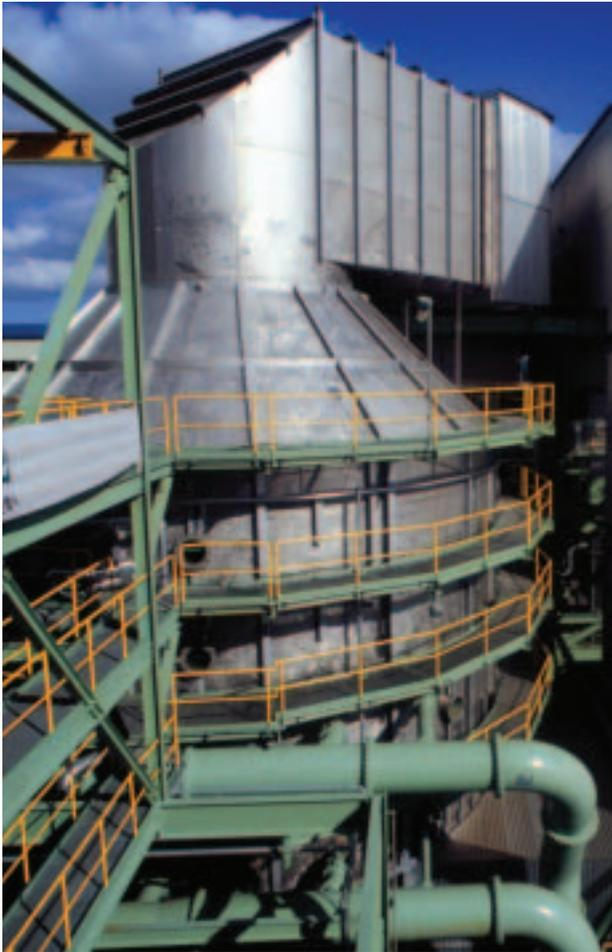
Pollution control equipment for coal fired electrical power generation plants use ATI's advanced specialty metals for Flue Gas Desulfurization (FGD) units.
