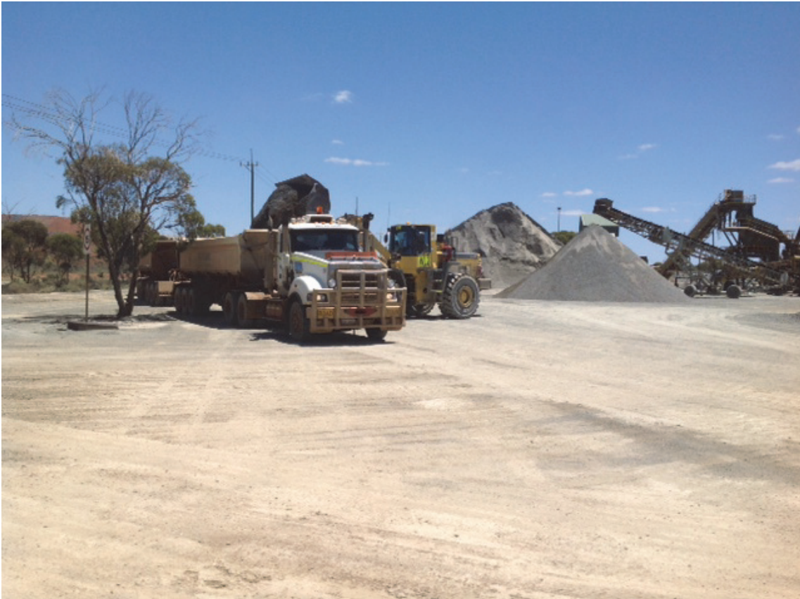
Figure 2 – Commencement of Crushing and Sampling - February 2016
