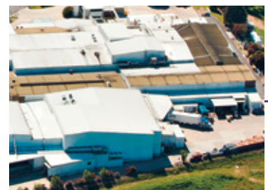
BEGA HEAD OFFICE AND PROCESSING & PACKAGING PLANT 23-45 Ridge Street Bega NSW 2550 Australia
