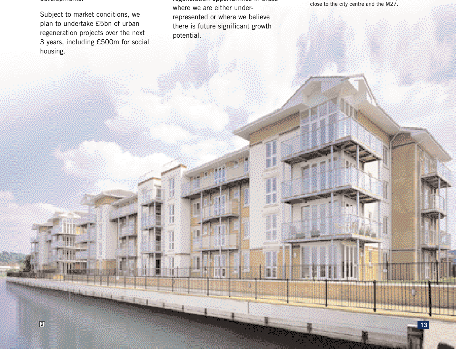
2 Clausentum Quay, Southampton. This spectacular development of 85 apartments is on a well-located waterfront factory site close to the city centre and the M27.
