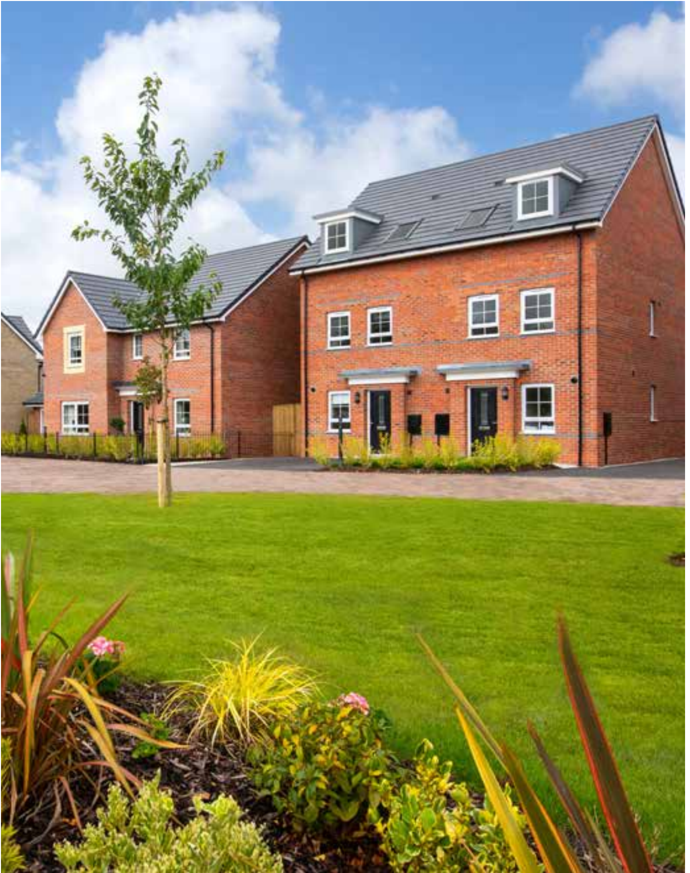
↓ Barratt Homes at Saviours Place, Stretton, Warrington.
