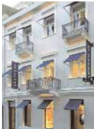
December saw the launch event for the opening of Burberry's first free standing store in Greece centrally located in a period building on the prestigious Voukourestiou Street in Athens.
