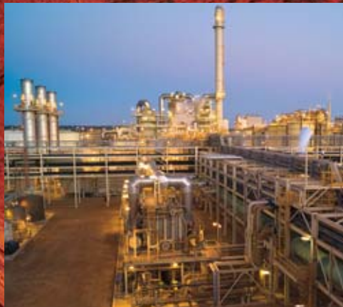
Ravensthorpe Nickel Operations, Australia
