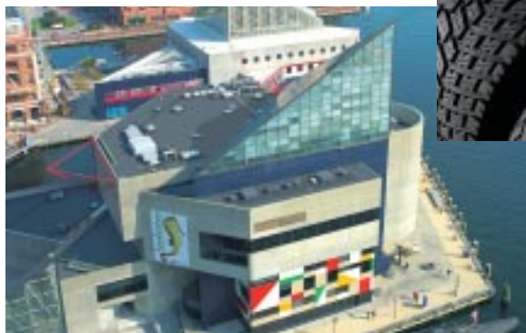
Carlisle SynTec roof on the Baltimore Aquarium in Baltimore, Maryland
