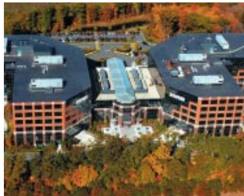
Carlisle SynTec's EPDM roofing system on the Staples Corporate Headquarters in Framingham, Massachusetts
