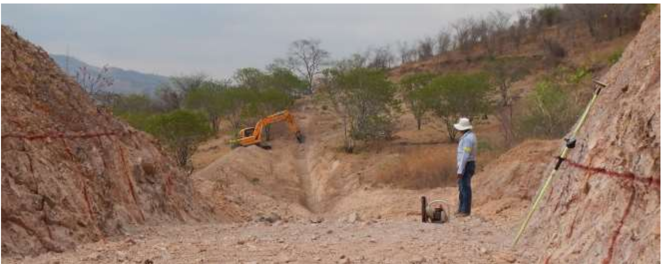
Figure 7. Trenching at Real de La Cruz core zone.
