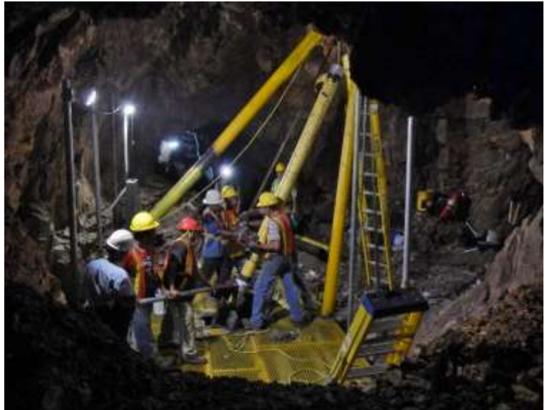
Figure 3. Installing a water pump in the historic La India Mine workings for the hydrogeology and mine dewatering testwork.
