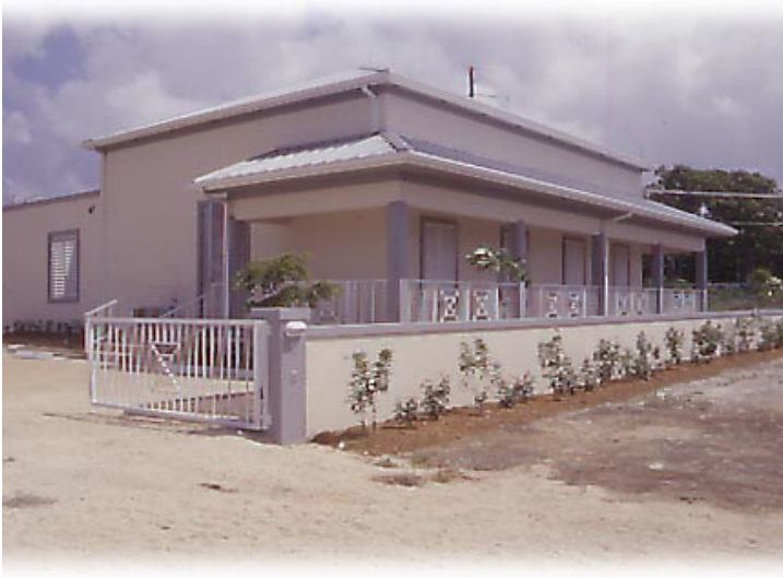
CUC commissioned its new 69KV South Sound Substation in November 2000. The substation was constructed by CUC's substation strategic alliance partner, ABB.
