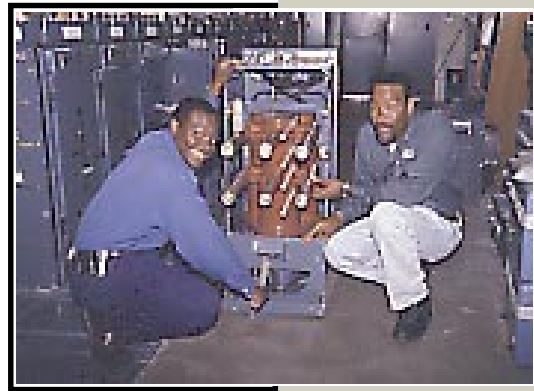
Earlton Bramble, Electrical Technician II, and Hinsley Hurlston, Industrial Electrician Helper.
