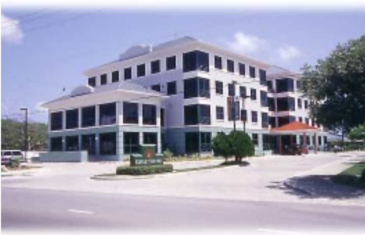
Cricket Square Phase II in George Town was completed in 2001.
