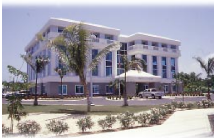
The 48,000-square foot BritCay House in George Town was completed in July 2001 and is one of several large commercial projects scheduled to come online in fiscal 2002.
