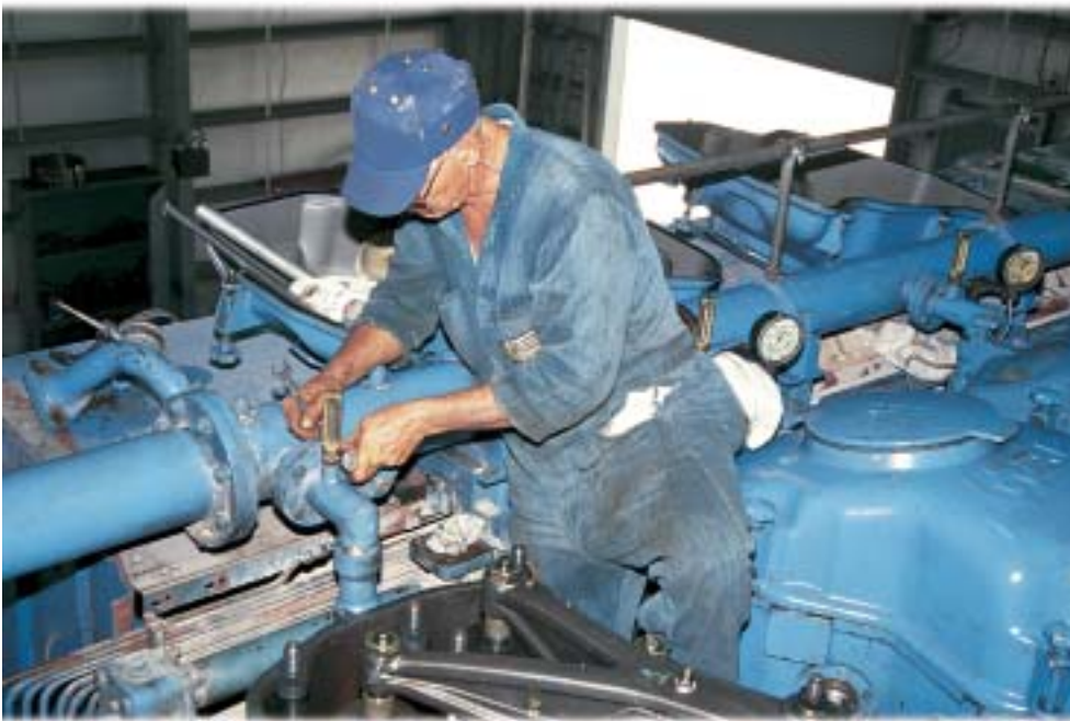
Eighteen-year employee Whitman Ebanks, Heavy Duty Mechanic, reattaches a dial after an overhaul on a generating unit. Part of the Company's Human Resources mission is to maintain its employer of choice status by providing career opportunities and competitive compensation while fostering personal growth and development.
