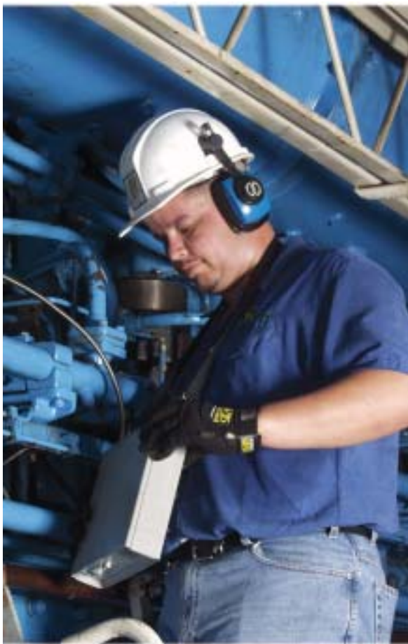
Jason Burke, Mechanical Technician, uses a pressure analyser to perform diagnostics on a generating unit. Jason, a CUC scholarship recipient, recently graduated from Texas State Technical College with Associate's Degrees, with high honours, in Industrial maintenance Technology and Facilities Management and Engineering.
