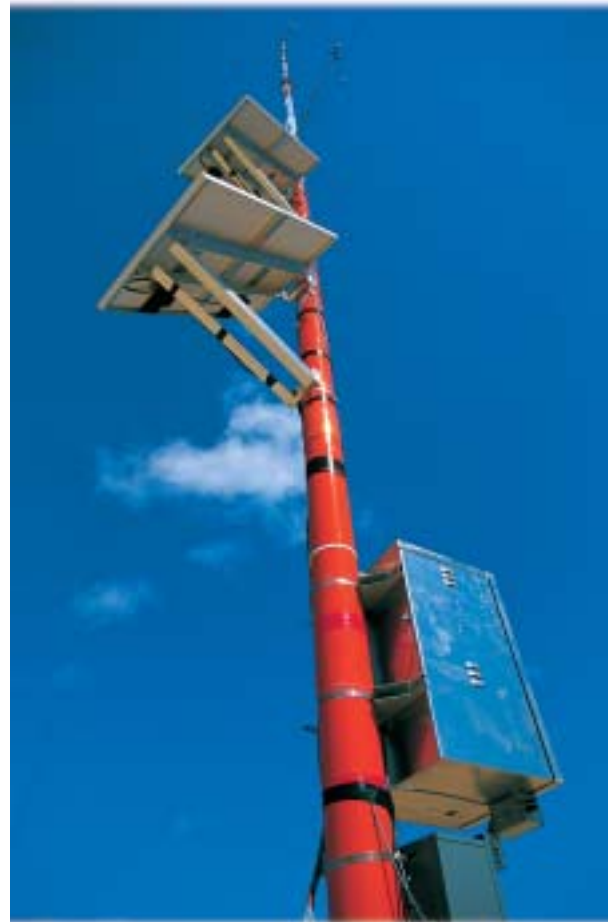
As part of its efforts to seek alternate sources of energy that are environmentally friendly, the Company erected two 170-foot wind-monitoring towers in 2002 to determine the feasibility of wind power.
