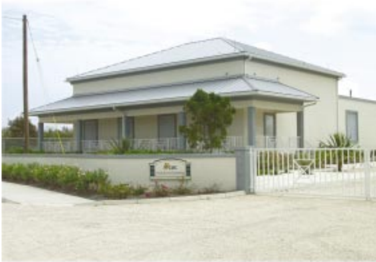
The 69 kV GIS Frank Sound Substation was energised in September 2002 to enhance the reliability of electrical service and to accommodate future load growth in the eastern districts. This substation is the second in a series of newly designed indoor substations.
