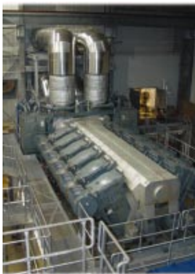
The newest 12.25 MW V48/60 MAN B&W diesel generating unit arrived in February 2003 and will be in full service by August 2003.
