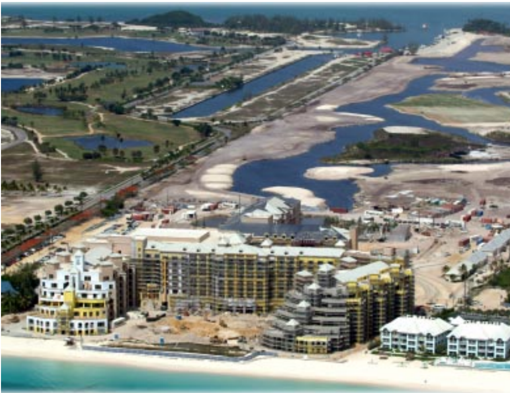
The 144-acre US$350-million Ritz-Carlton on world-famous Seven Mile Beach houses 69 luxury beach-front residences as well as a hotel section which is adjoined by an elevated walkway above West Bay Road. The 18-hole Greg Norman-designed golf course stretches from the rear of the hotel to the North Sound. The resort is scheduled for completion in December 2004.
