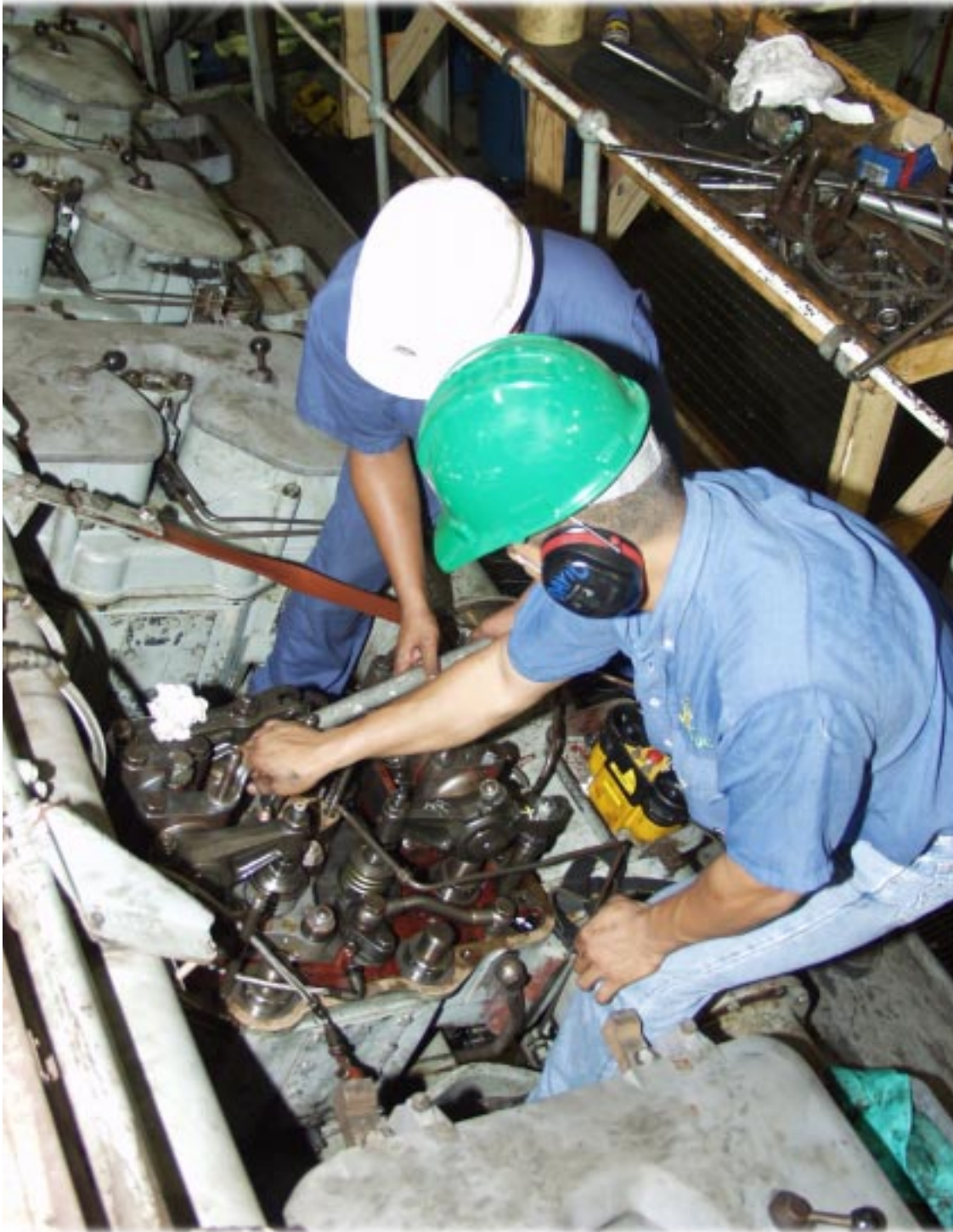
Kevin Winton and Dario Mayorquin from the Mechanical Maintenance Department complete maintenance on one of the Company's generating units. All generating units undergo a thorough maintenance schedule to ensure maximum efficiency.
