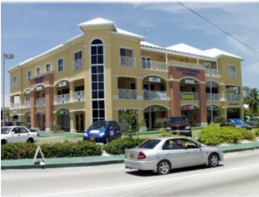
The recently completed 22,000-square foot Centennial Towers is West Bay's largest and most recent retail shopping and office complex. The Towers' residents include numerous small businesses as well as outlets for established businesses in George Town determined to cater to customers' needs in the outer districts.
