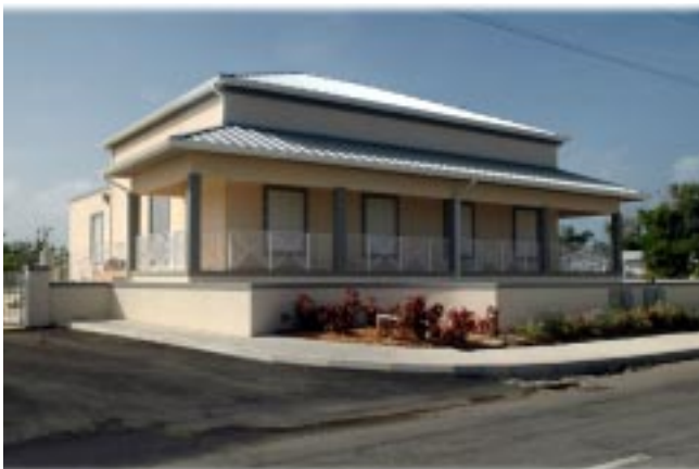
The 3,250 square-foot Hydesville Substation in West Bay, the fourth in a series of indoor substations, was commissioned in April 2005. The new substation houses four new distribution feeders which enhances reliability of electrical service in West Bay.
