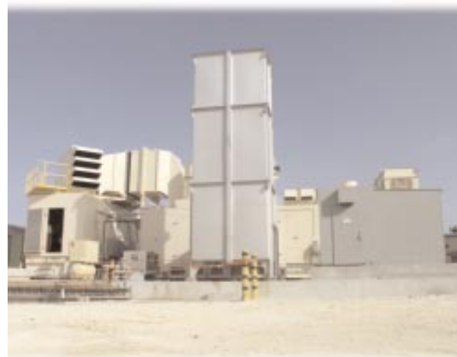
The newly installed 8.4 MW gas turbine was assembled during March and April 2006 and is in the final testing stage. CUC’s newest addition is scheduled to be commissioned in July 2006.
