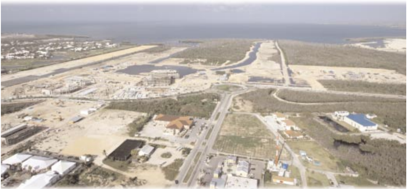
An aerial view of the 300-acre Camana Bay development off West Bay Road shows construction work on the Town Centre, which will house shops, restaurants, a cinema and school among other Island-oriented attractions. Once completed, Camana Bay will stretch from Seven Mile Beach in the west to the North Sound (shown at top) in the east, incorporating offices, residences, recreational areas, a harbour, beach access and an abundance of native vegetation.
