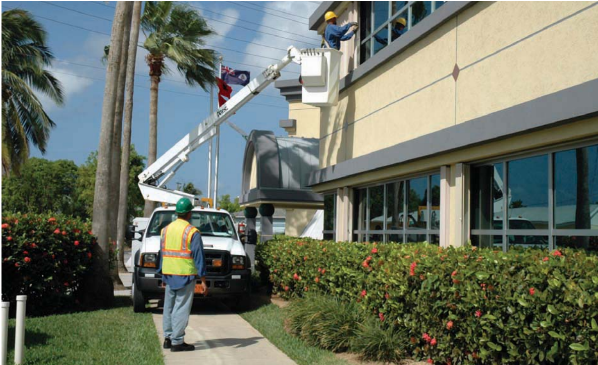
Each year, CUC conducts a hurricane drill prior to the beginning of the Atlantic Hurricane Season, which runs from June to November. One of the primary focuses is the protection of the Administration Building whereby members of the Line Operations team inspect the hurricane shutters.
