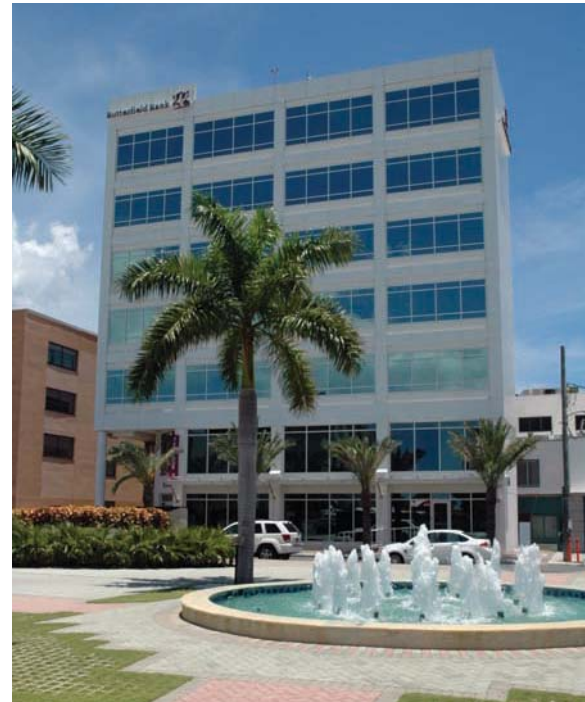
The seven-storey Butterfield Bank building, located in central George Town, the capital, was completed in May 2007.
