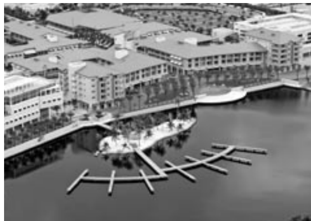
The next phase of the 500-acre Camana Bay development includes an estimated additional 25,000 square feet of commercial space.
