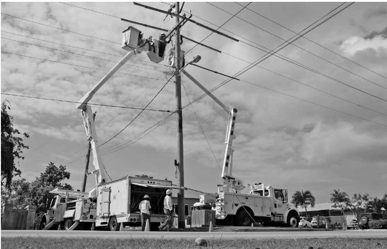
In 2012, the Company embarked on a number of major transmission and distribution projects including the removal of a large section of distribution lines and hardware around the Island's airport and the subsequent re-routing of service through newly constructed poles and lines.
