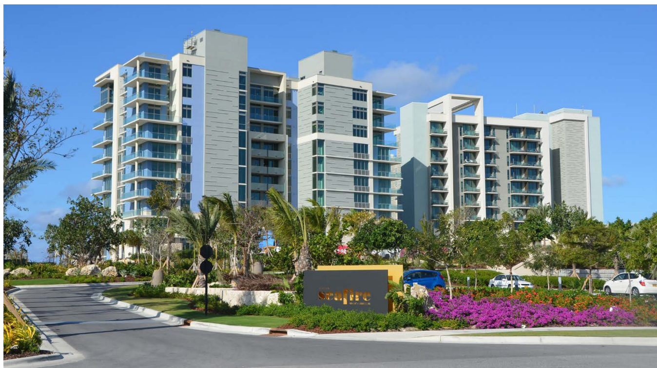
The Kimpton Seafire Resort and Residences was completed in November 2016.
