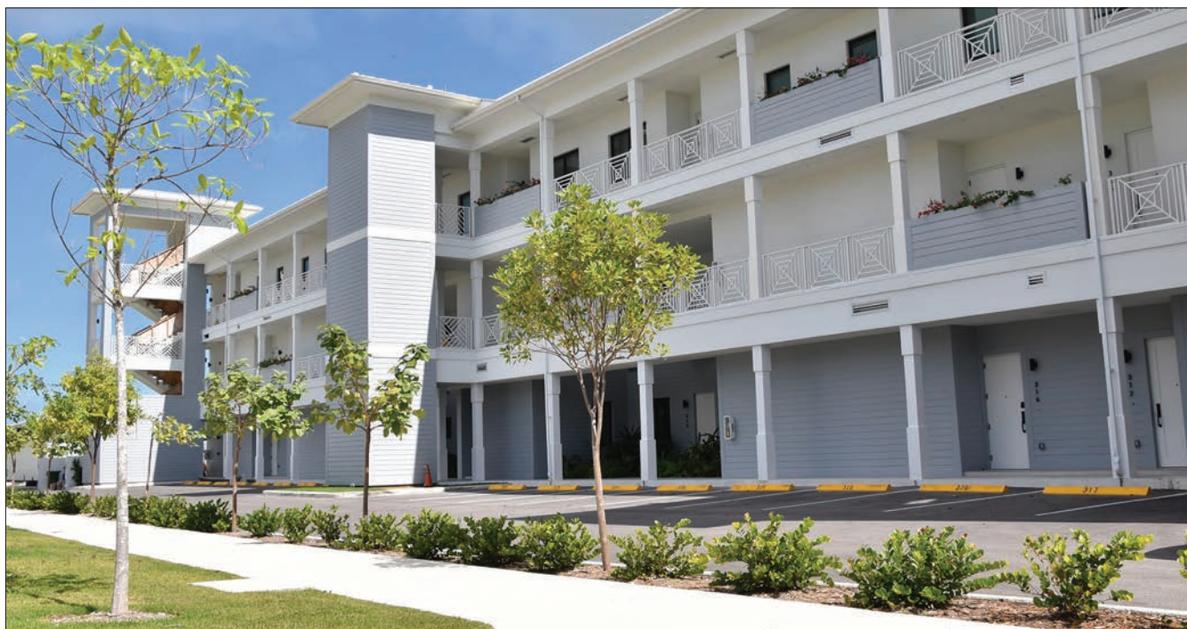
The COVID-19 pandemic affected the construction industry on Grand Cayman during 2020 and 2021 although several large developments, such as OLEA at Camana Bay, which will eventually comprise condominiums, townhomes and duplexes when completed, continued construction efforts throughout the pandemic. Phase 1 of OLEA was completed in June 2021.
