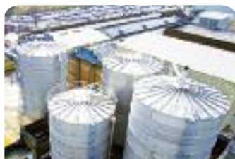
The new stock preparation plant was a major part of the investment to modify New Thames Mill at Kemsley.
