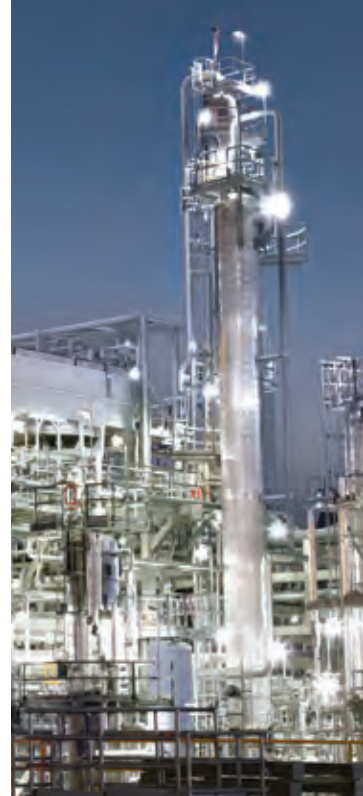
The acquisition of the El Dorado refinery more than doubled Delek US' combined production capacity
