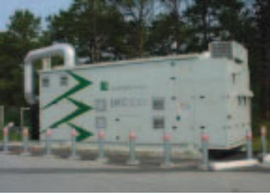
This DFC300A power plant at the Coast Guard Air Station Cape Cod in Massachusetts provides heat and power for the emergency personnel using the facility's barracks.
