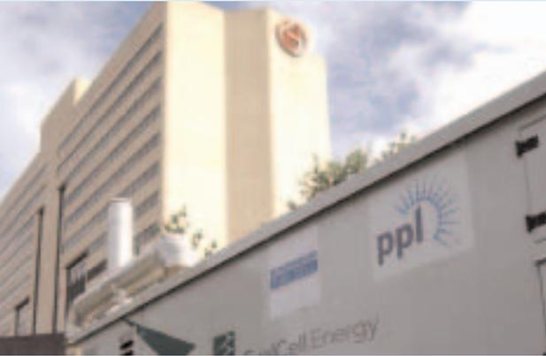
The Sheraton Edison (top) and the Sheraton Parsippany (bottom) each have a DFC300A power plant that provides the base load electricity requirements and 25 percent of the hot water needs for these New Jersey suburban hotels.
