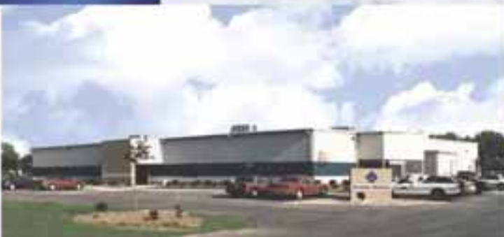
Located in Grant County, Indiana, Franklin's Electronic Technology Center is dedicated to the production of electronic controls and drives.
