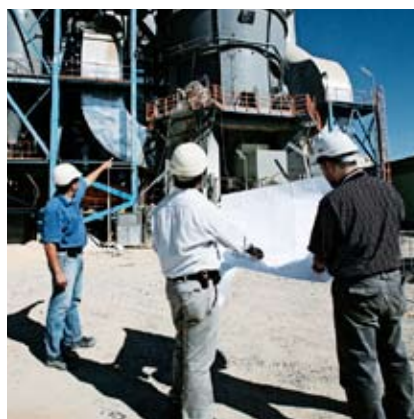
At the construction site of a new FLSmidth cement plant in the Middle East, the packing plant and the ATOX raw mill department are being inspected.
