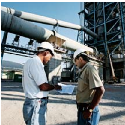
Checking some installation details.
