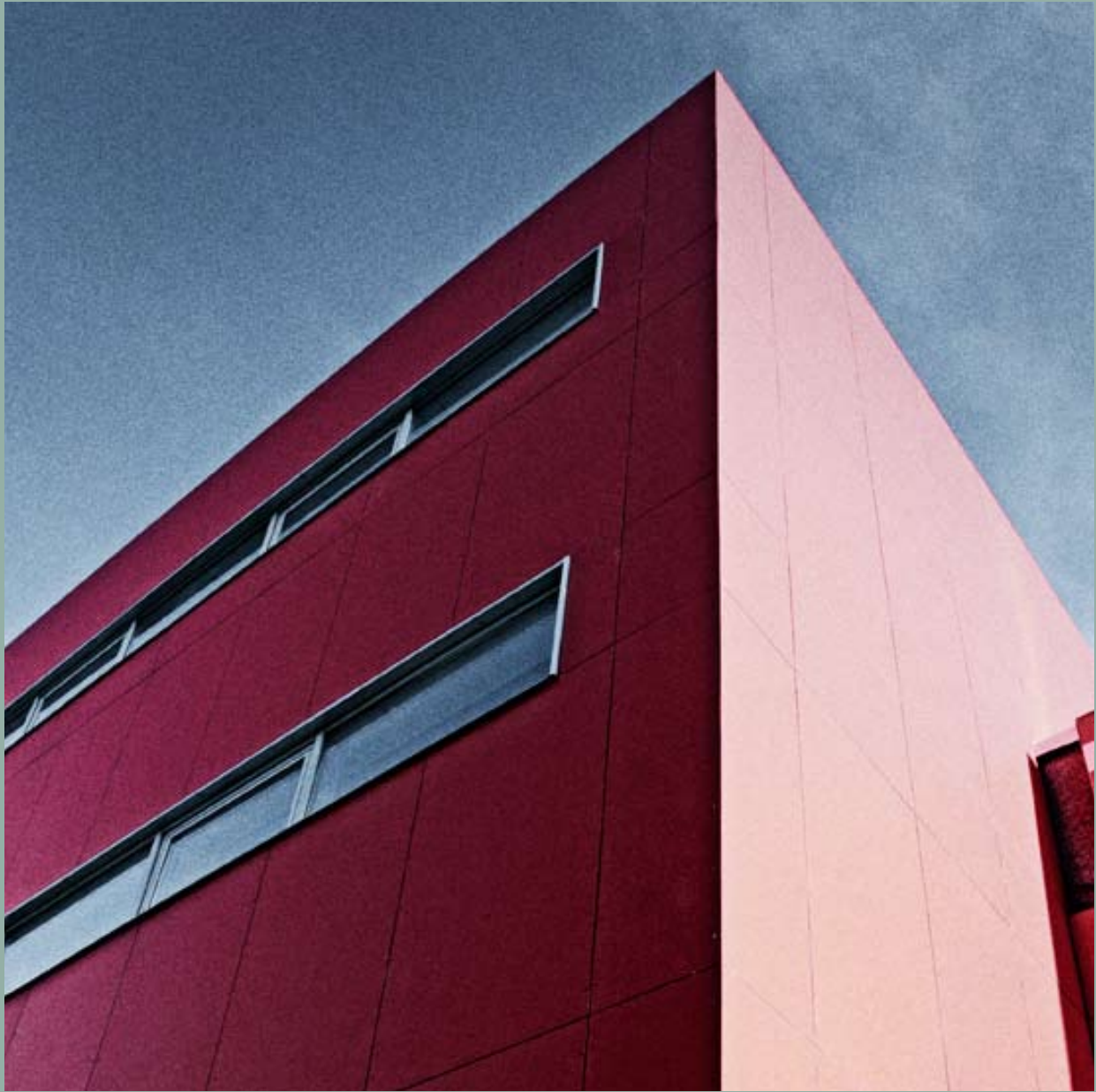
Cembrit produces and markets a wide range of fibre cement products in Europe. Pictured here are flat sheets for external cladding of facades.
