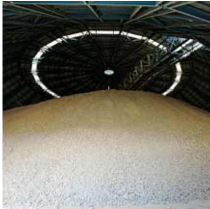
FLSmidth MVT circular raw material homogenising store.
