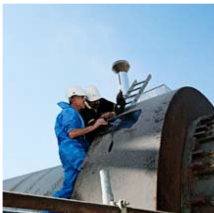
FLSmidth inspectors check cement kiln tyre, cement clinker conveying equipment and storage silo.
