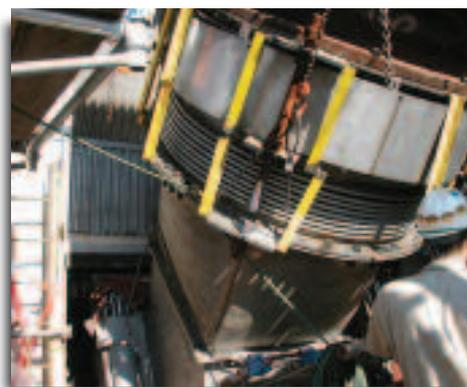
At ExxonMobil's refinery in Baytown, Texas, Fluor provides EPCM services for a variety of clean fuels projects to support the client's emission reduction goals. Pictured above, a new refractory lined expansion joint being installed upstream of a new Ultra Low NOx burner as part of the NOx Reduction project at the refinery.
