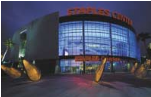
The Staples Center in Los Angeles, California, a $400m sports and entertainment venue protected by 1,000 Apollo fire detectors.
