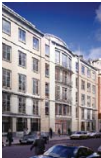
HAMMERSON'S NEW HEAD OFFICE AT 10 GROSVENOR STREET IN LONDON, W1.
