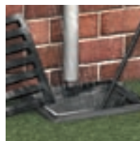
Unblock drain by jetting
