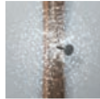
Repair pipework following a DIY accident
