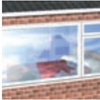
Replace broken window
