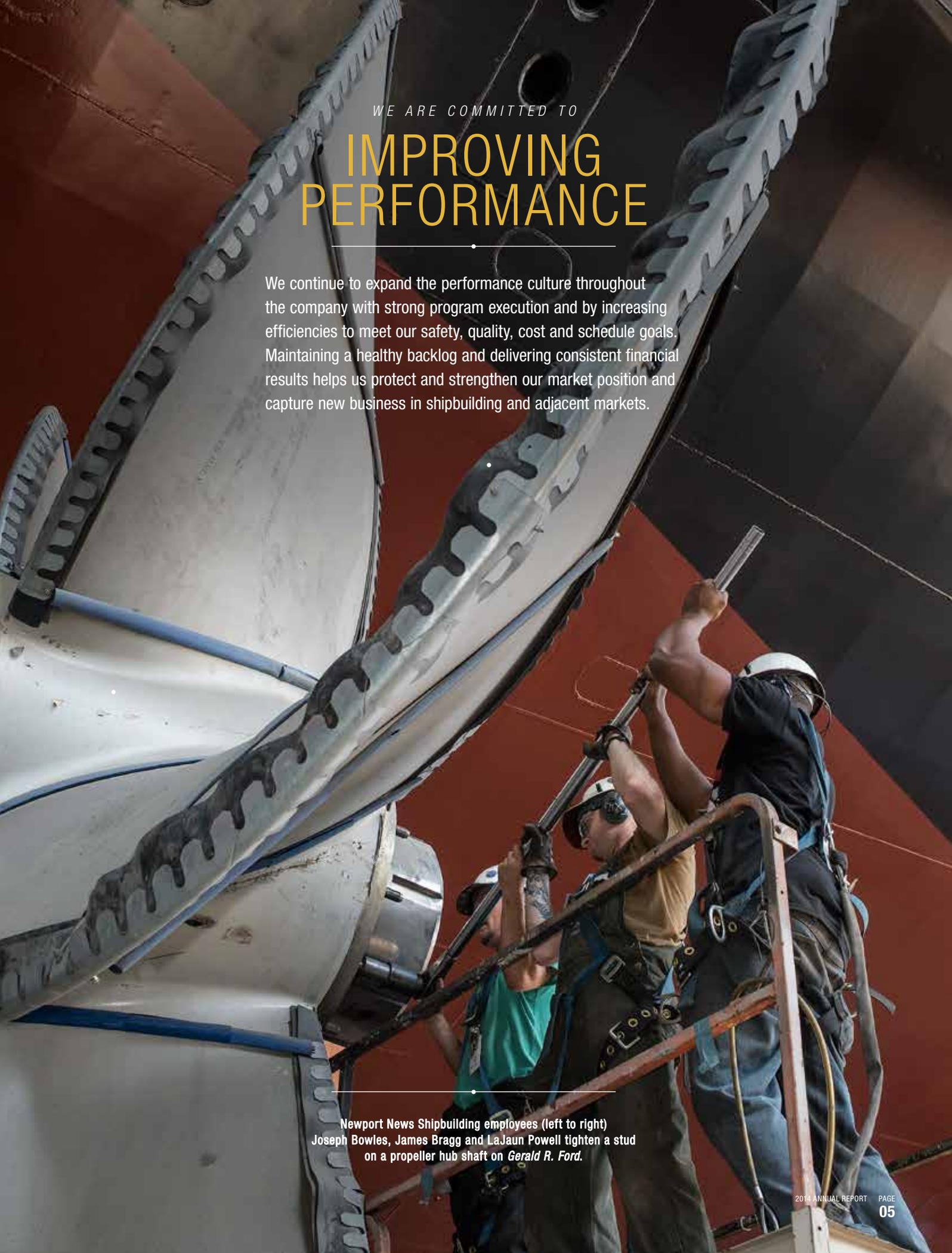
A low-angle photograph of three shipbuilding workers on a wooden scaffold. They are working on a large, metallic propeller hub shaft. The workers are wearing hard hats, safety harnesses, and work clothes. The background is a large, reddish-brown structure, likely part of the ship's hull. The lighting is bright, highlighting the metallic surfaces and the workers' efforts.
