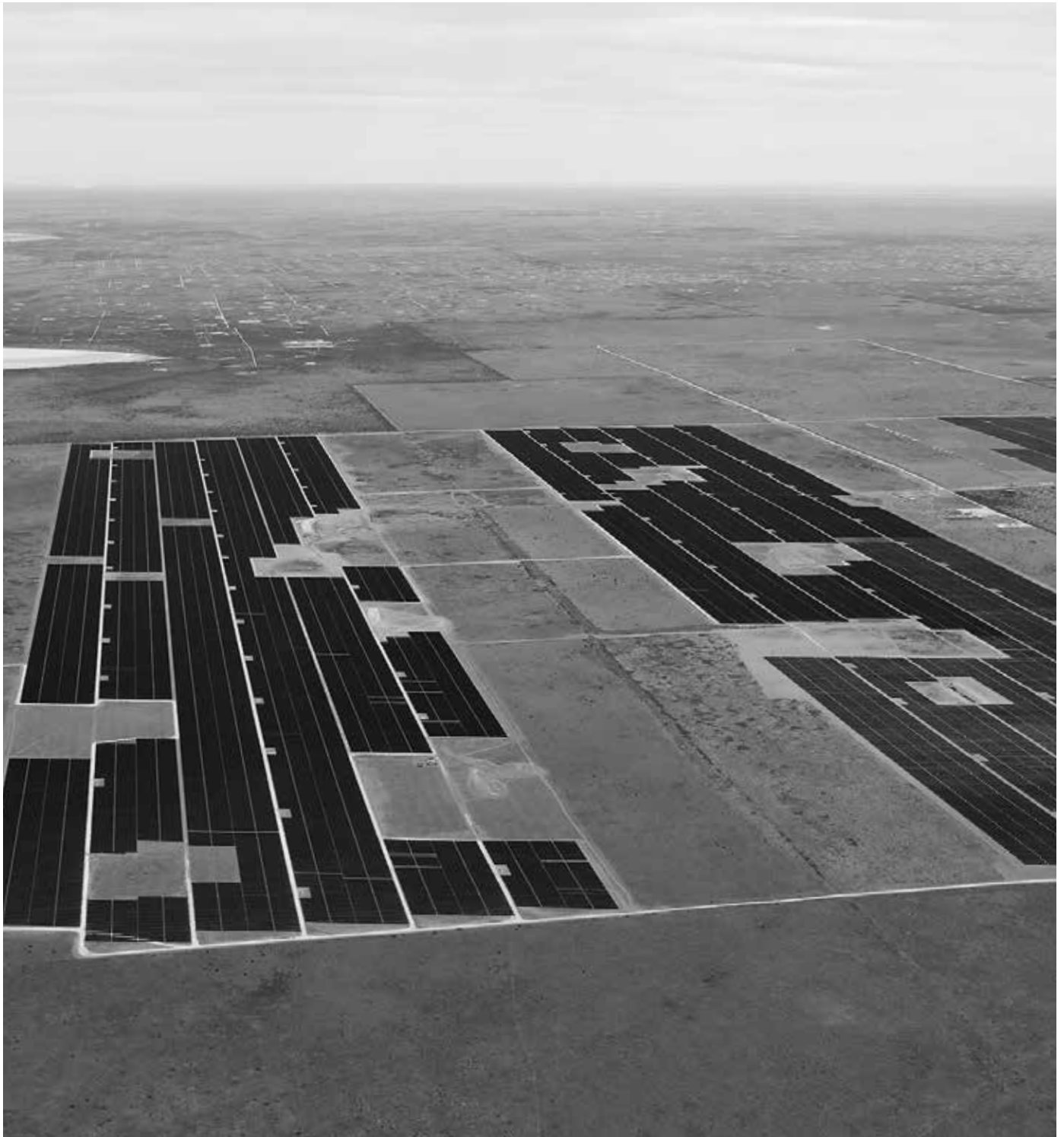
Prospero Solar project, Texas, USA.
