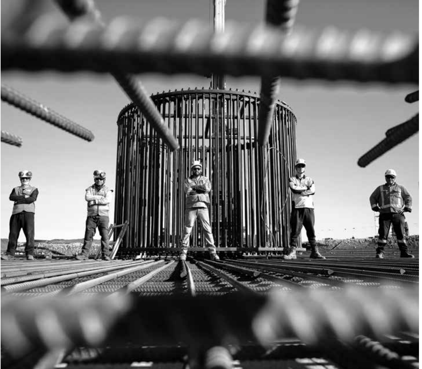
Waipipi wind farm construction workers social distancing under Level 3 restrictions.
