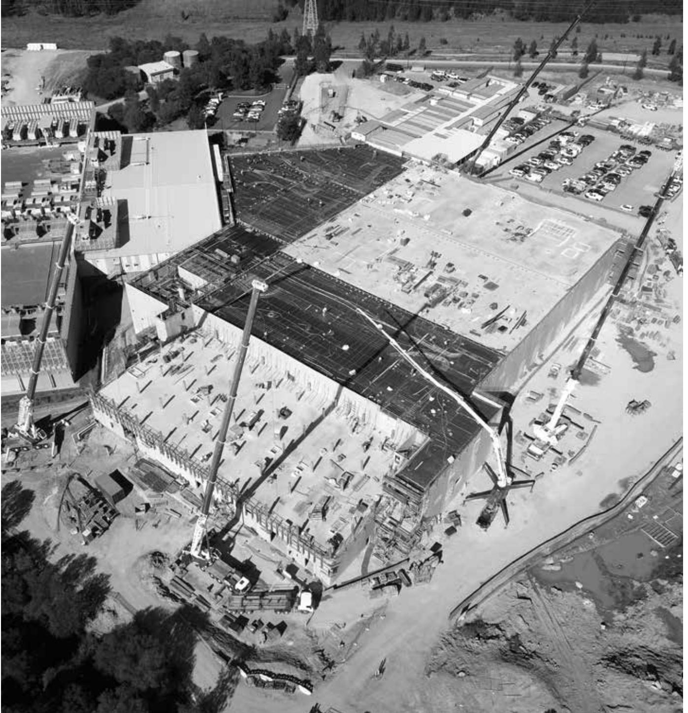
Construction of CDC's Eastern Creek 3 data centre, Sydney.
