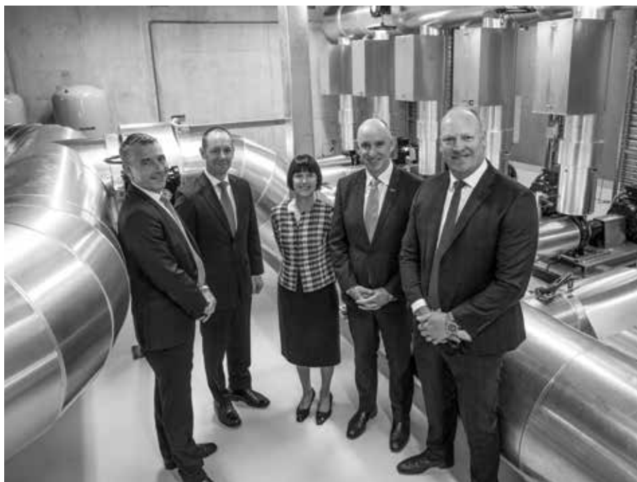
The CDC Fyshwick 2 facility opening, December 2019. From left to right: Brett Chenoweth: Chairman, CDC Data Centres, Randall Brugeaud: Chief Executive Officer at the Digital Transformation Agency, Renee Leon: Secretary of the Department of Human Services, Hon. Stuary Robert MP: Minister for National Disability Insurance Scheme and Greg Boorer: Chief Executive Officer & Founder, CDC Data Centres.
