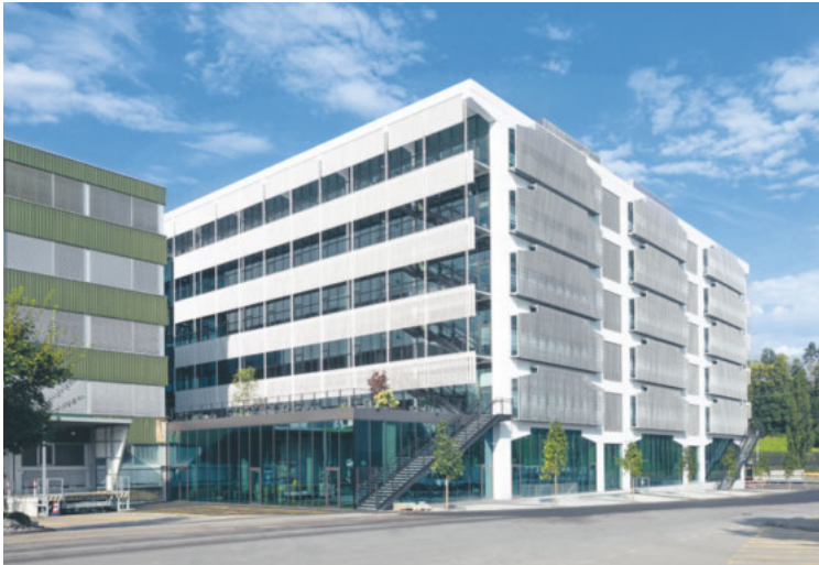
For its new headquarters building in Dierikon, which was occupied in 2020, Komax opted for a low-tech, climate-friendly approach.
