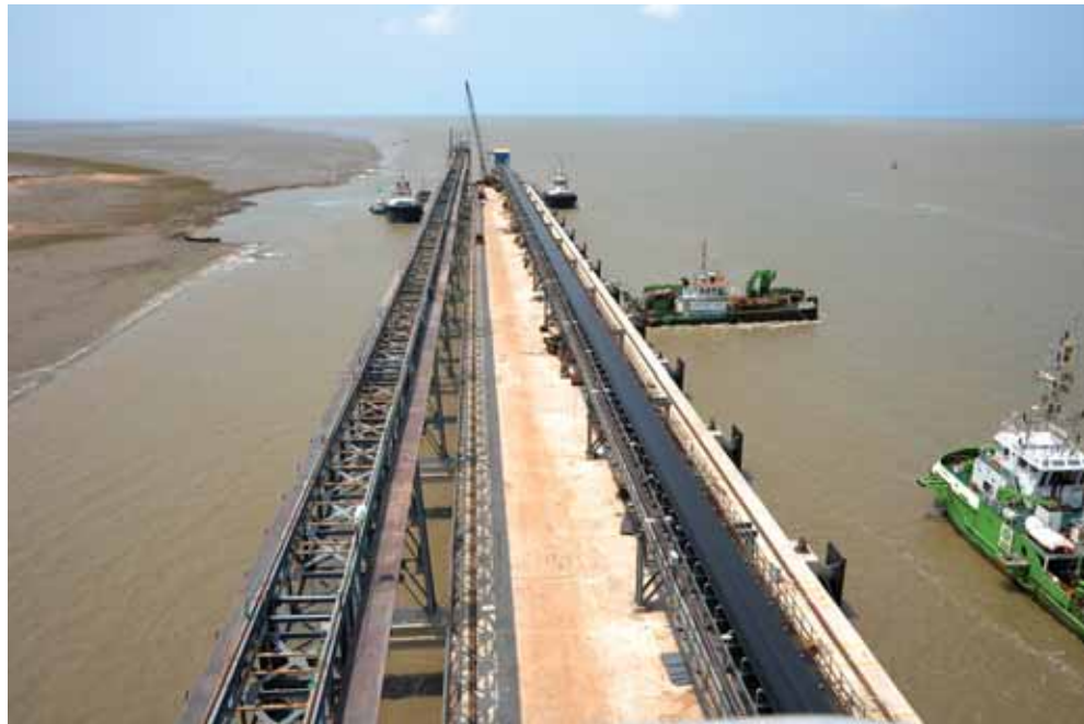
Port at Dhamra on India's east coast developed by L&T in collaboration with the Tata Group. L&T is carrying out complete civil, electrical and mechanical construction for this major port complex.
