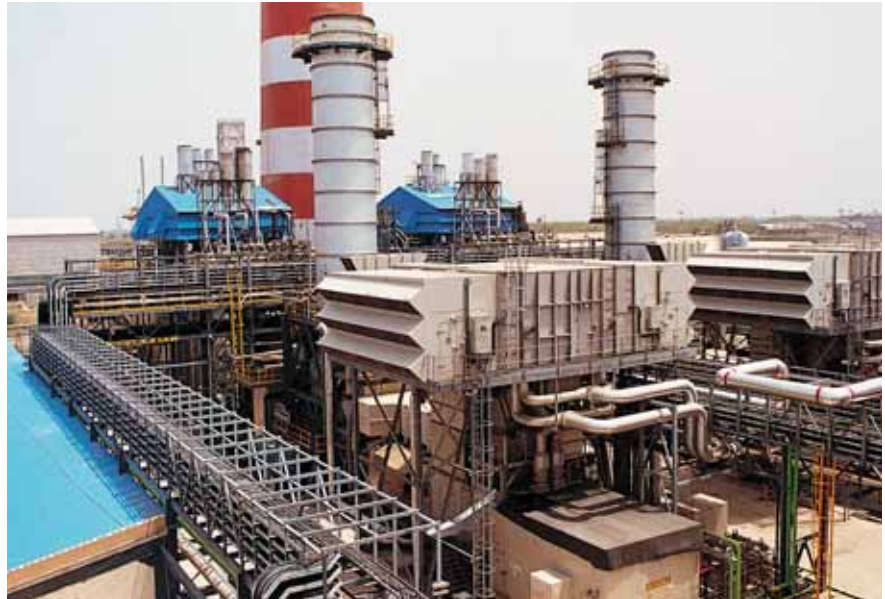
90 MW co-generation power plant at IPCL, Gandhar.
