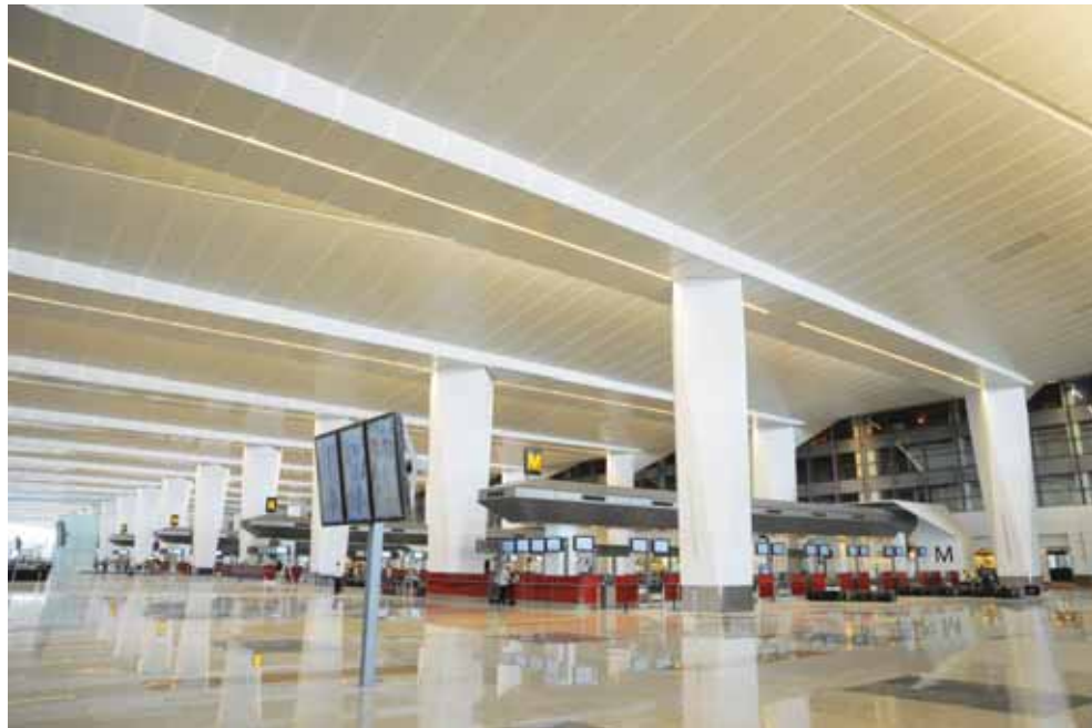
Terminal III of the Indra Gandhi International Airport, Delhi. L&T is driving the airports revolution in India, building virtually every major new international airport in the country.
