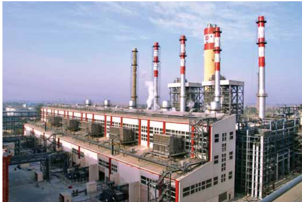
Power plant executed by L&T on an EPC basis at the complex of Indian Oil Corporation in Panipat.
