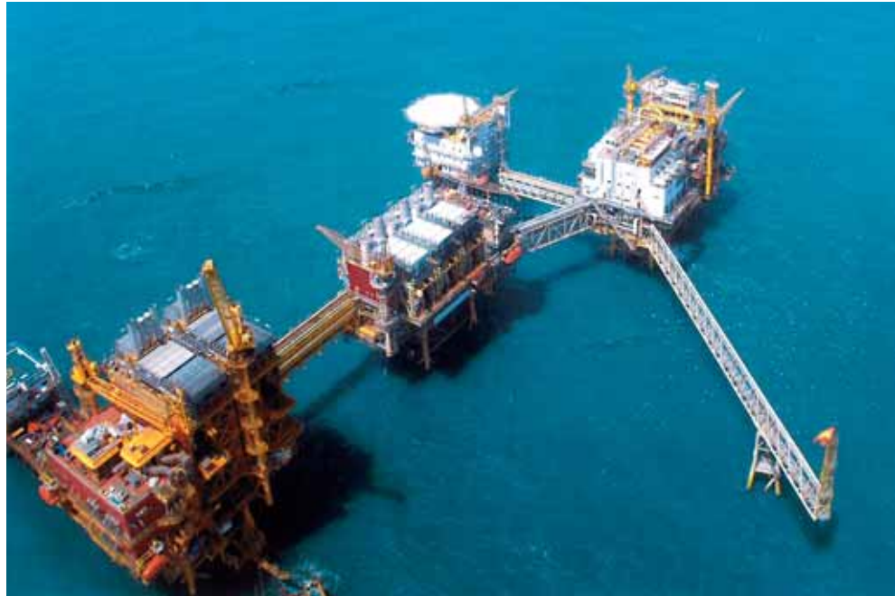
BCP-B2 Process Platform and Well-head Complex connected to the pre-existing BPB Complex for Oil & Natural Gas Corporation, located in the Bassein Gas Field, approx. 80 km north-west of Mumbai.
