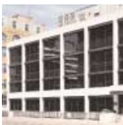
203/5 Blackfriars Road, London SE1
