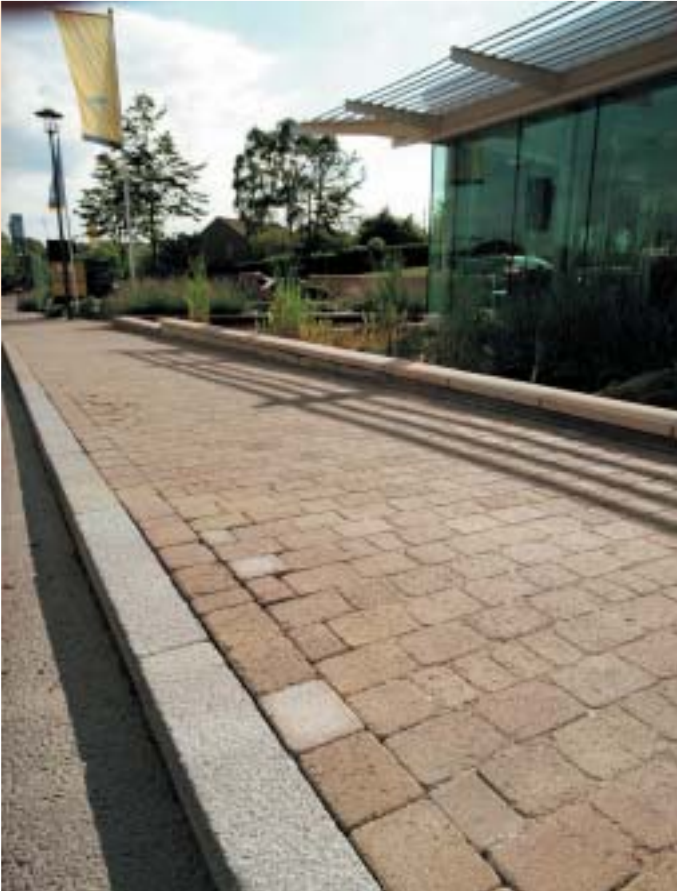
Port Marine, Portishead. Tegula Block Paving
