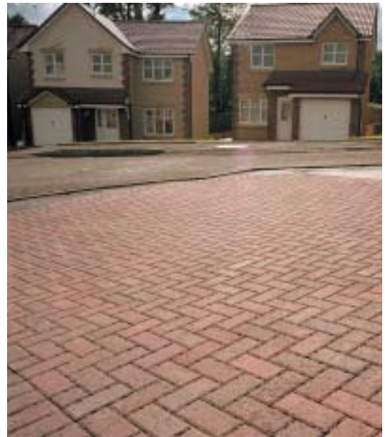
Priora block paving. Sustainable Urban Drainage System
