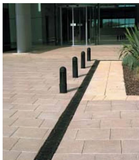
Perfecta paving & Birco linear drainage. Chineham Court
