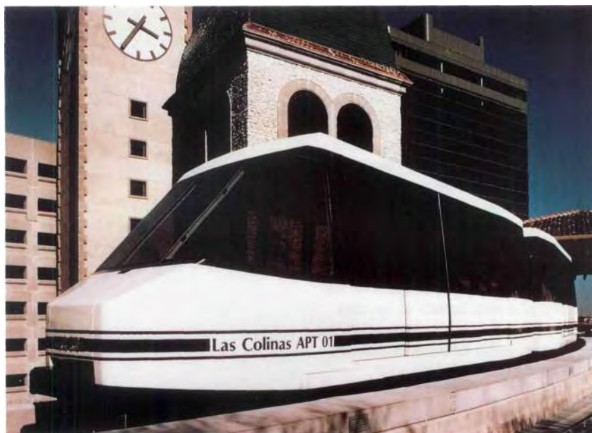
Easily integrated transport systems already exist: the Area Personal Transit System in Las Colinas, Texas, USA
