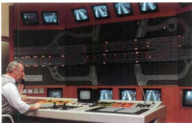
Supplied by AEG: the central operating and control unit for monitoring and regulating traffic flow in the Ems Tunnel
