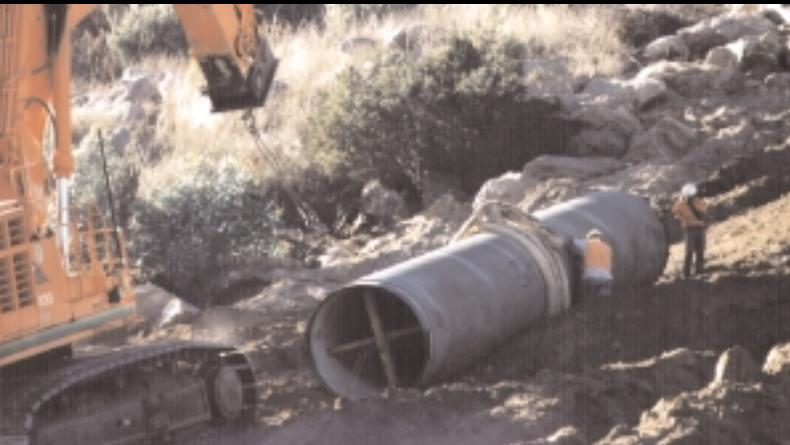
Mortar coated steel pipe can tackle the most demanding handling and installation environments.
