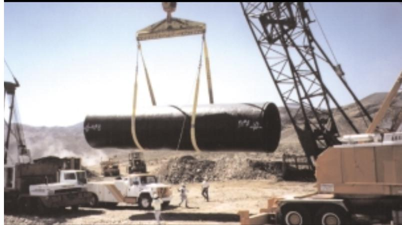
108" welded steel pipe with mortar coating was the choice of this pipeline serving the growing Las Vegas, Nevada area.
