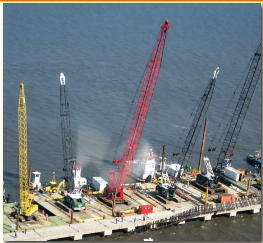
Floating cranes all in a row tower over the barren deck of the Lake Pontchartrain trestle following Hurricane Katrina. As seen at lower right, the cranes recovered 4.8 miles of track from the lake and lifted it back onto the bridge.
