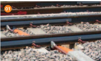
**01 Remote condition monitoring measures and records the impact of trains on the rails. This allows us to identify defective train wheels and overloaded axles which can then be maintained to reduce track damage.**
