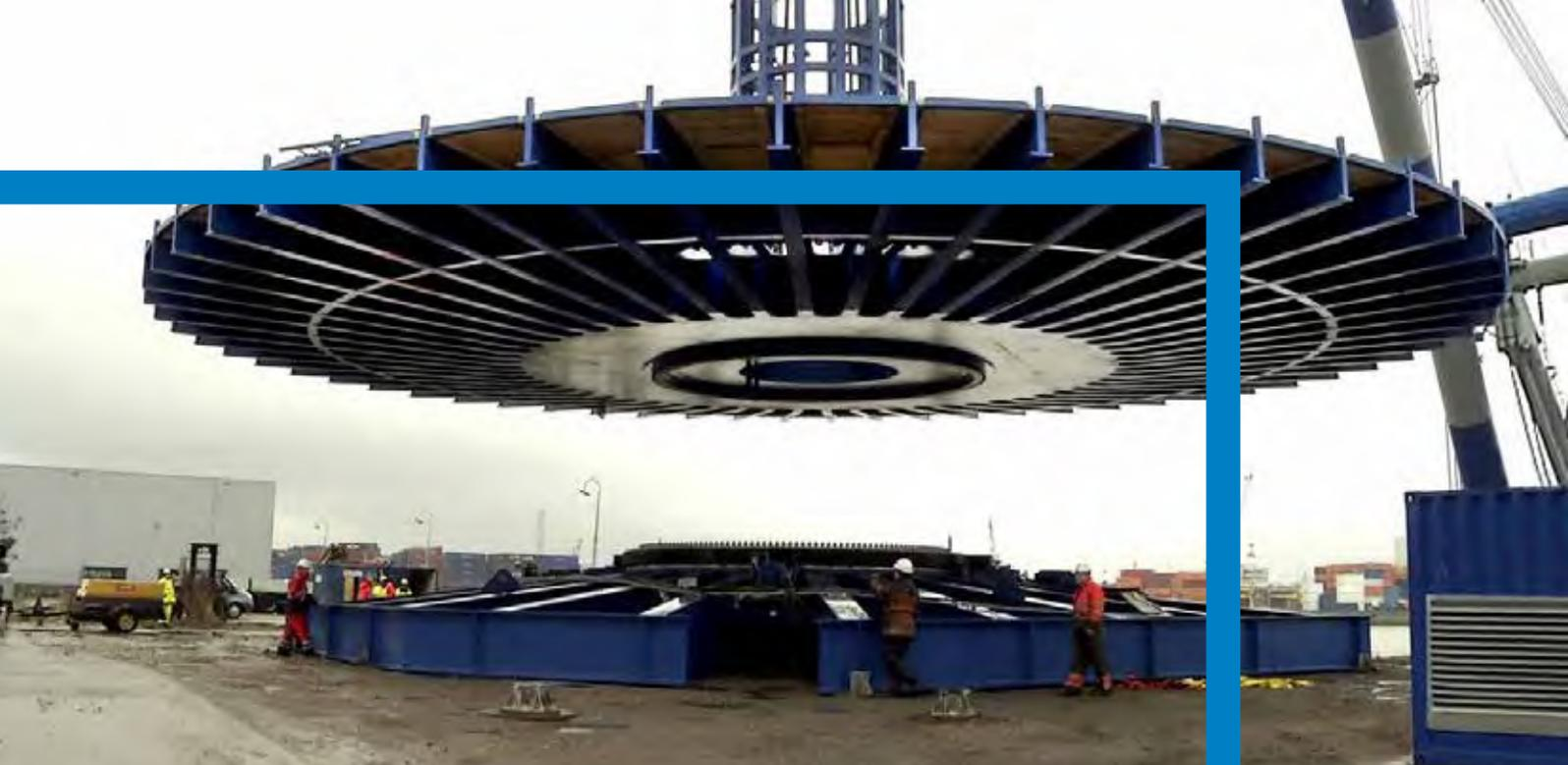
Installation of the turntable at the transshipment and storage terminal in Rotterdam which significantly increases the storage capacity for submarine cables.
