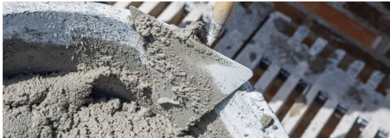
Detail from PensionDanmark's construction site at Islands Brygge
