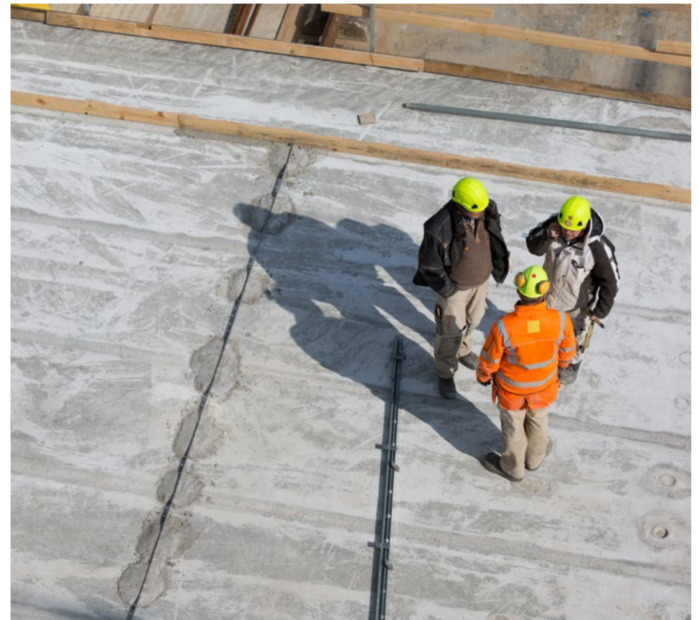
PensionDanmark's construction site at Islands Brygge
